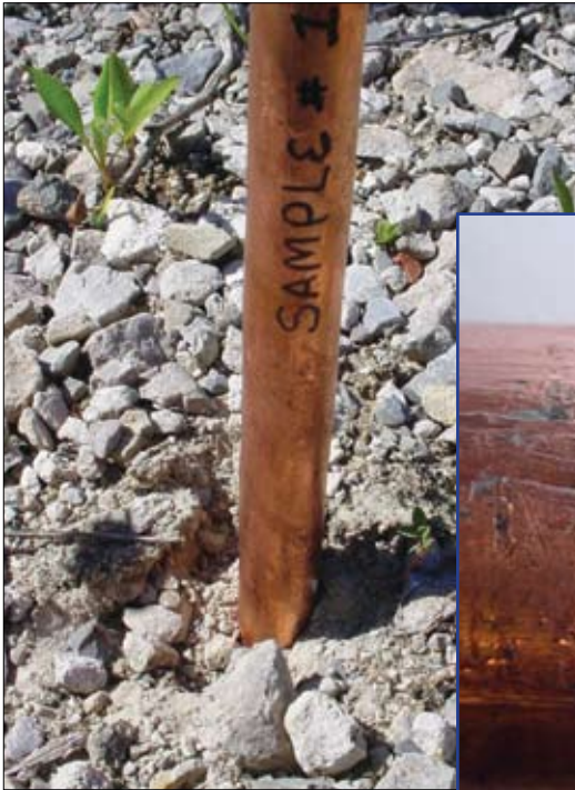
Photo 1(a). Example of driven ground rod
